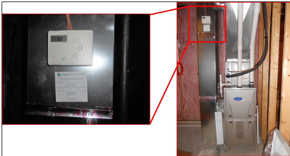
P4. If you have ventilation air intake at the furnace, it will look something like this. You will need to check your user's manual to change its settings.
