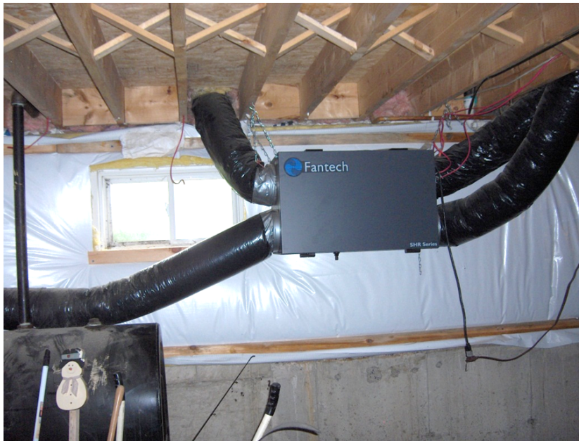
P5. This is a common appearance of a heat recovery ventilator (HRV). You will have to check your user's manual to set it.
