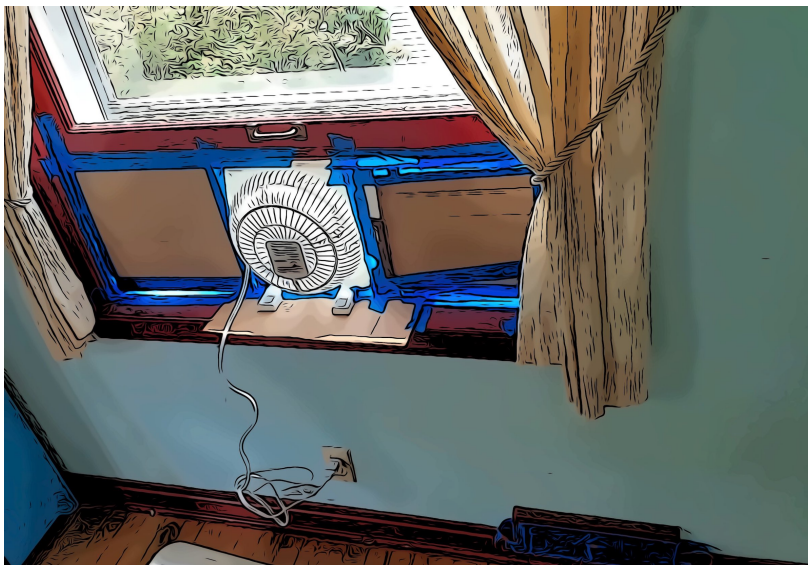
Photo 5. Fan mounted in window to blow outdoor air into the room, with window sealed except where the fan is.
