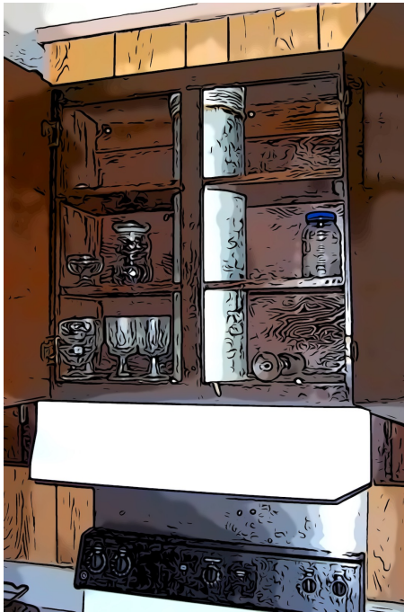
Photo 4. Kitchen range hood, showing duct to outdoors. Range hoods without a duct do not increase ventilation.
